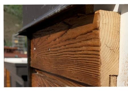
**NOTE:** Not sealing these cuts, rips, holes, etc, will allow your siding to absorb water, and potentially cause the color/finish to fail and "bleed."
