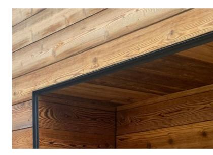
**NOTE:** Only reseal areas that NEED resealing. If you inspect areas of your siding (such as north/ northeast facing), and the finish appears smooth/solid, you do not need to refinish. Adding unnecessary additional layers of oil coating will cause your siding to appear "shiny," with a plastic- like façade.
